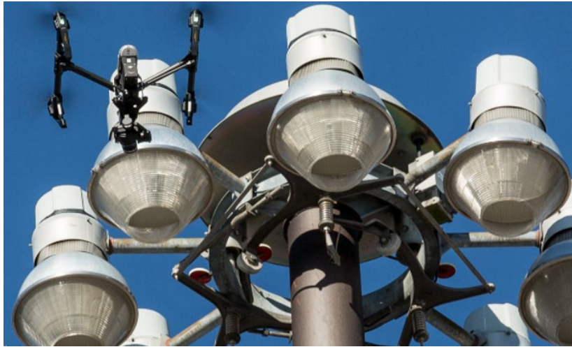
Figure 1. UAS Inspecting HMLP. Source: NJDOT
