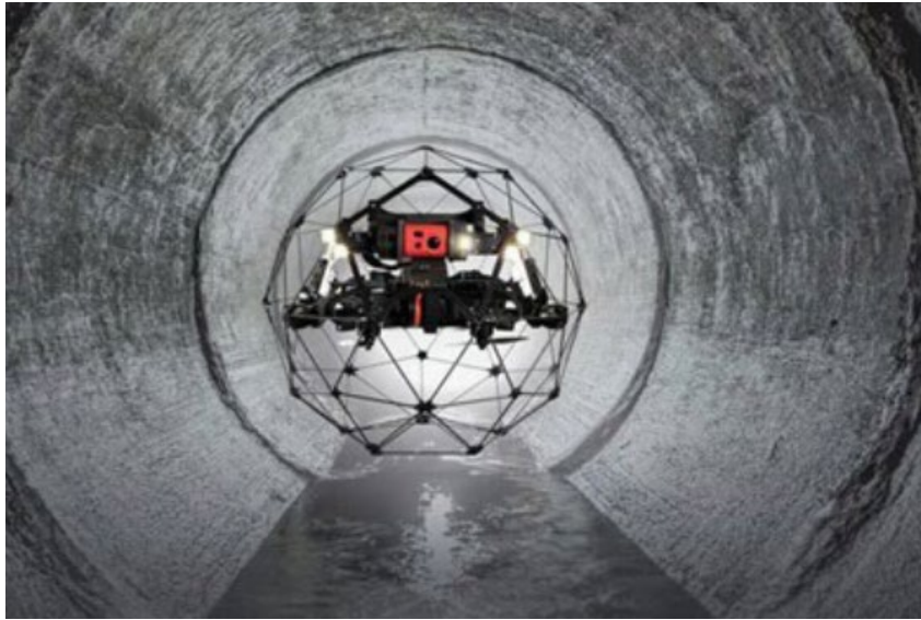
Figure 5. UAS Inspection of Large Pipe. Source: MDOT
