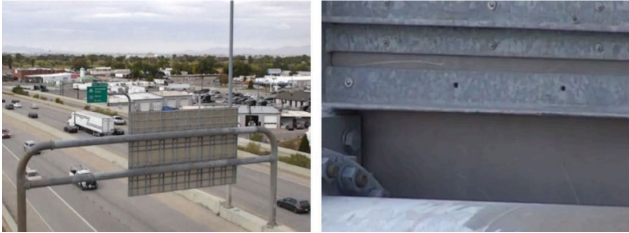
Figure 6. UAS Overhead Sign Inspection. Source: UDOT
