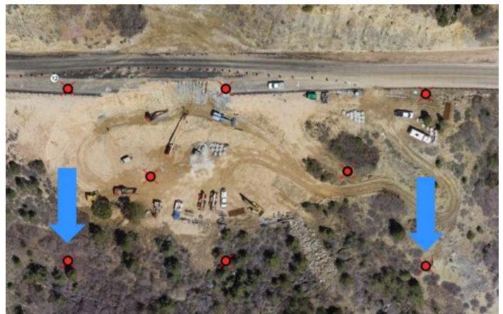
Figure 9. GCPs placement (Image courtesy of UDOT)
